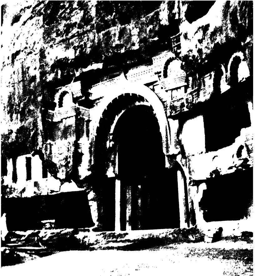
Facade of Chaitya Hall, Bhaja, Western India, 2nd century B.C. (Courtesy, Department of Archaeology, Government of India)
